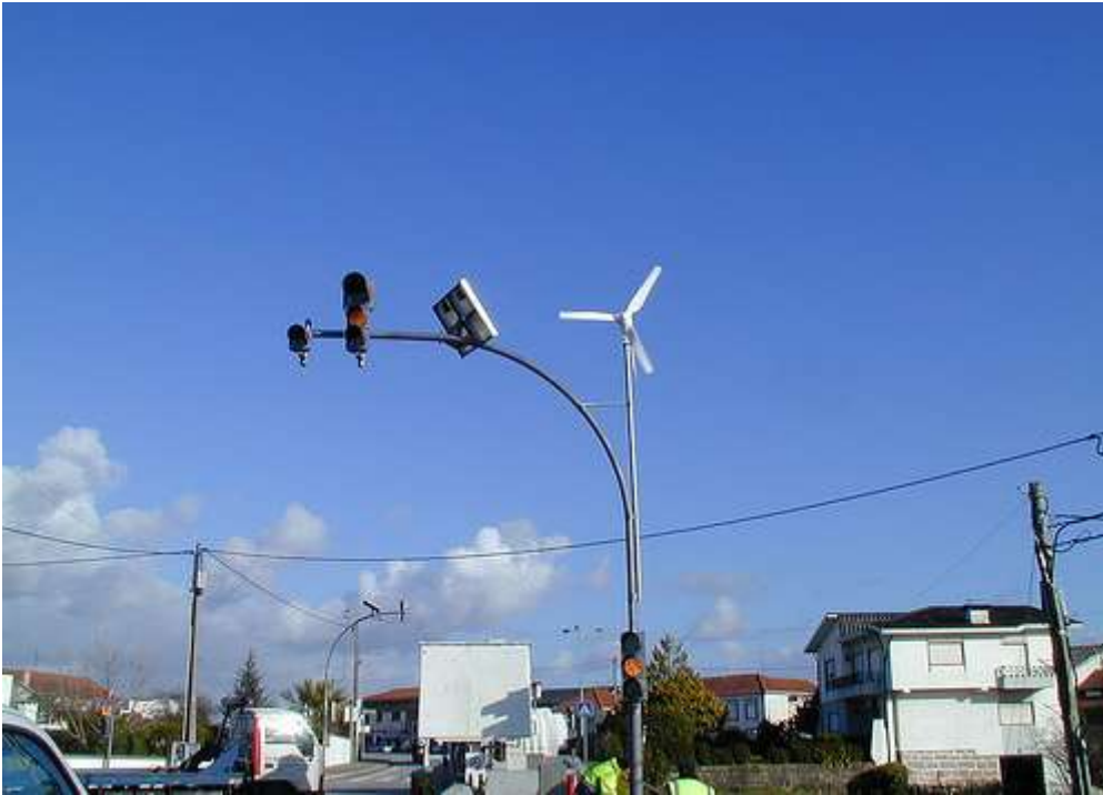
Fig. 3 - Solar and wind powered microwave system (courtesy of Eyssa-Tesis Portugal).
